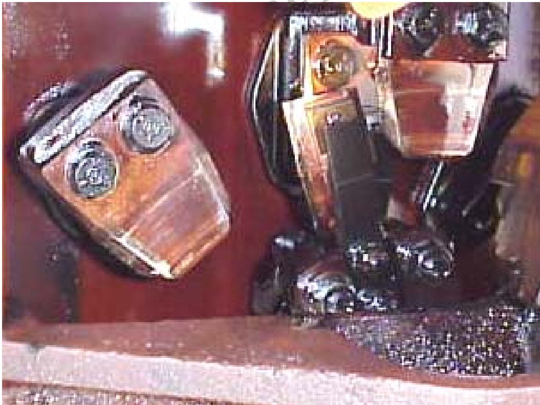
Normal Wear on Moving Contacts FIGURE 3
