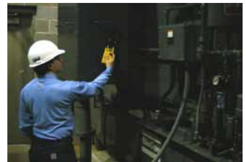
EMI Diagnostics provides a broader view of system defects including stator winding partial discharge.
