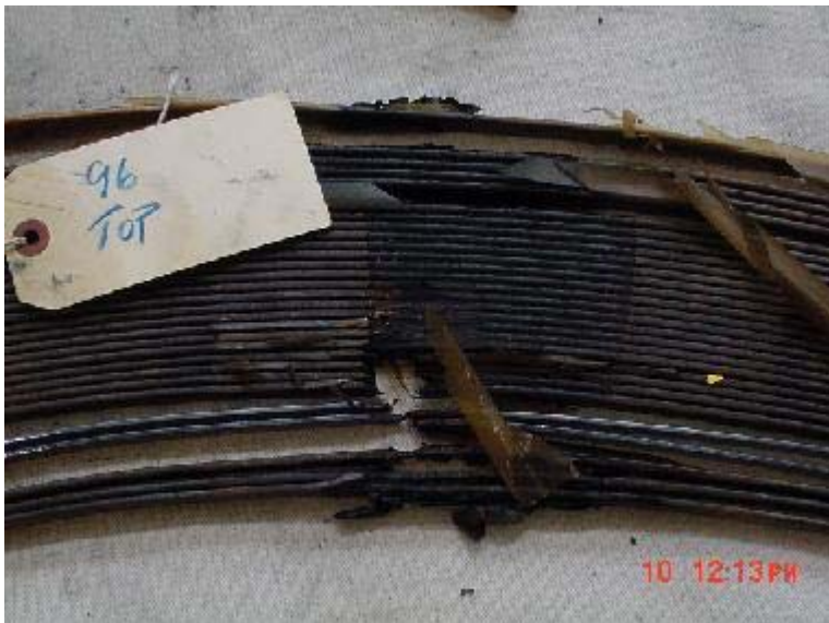
Figure 2: Evidence of Discharge Activity on a Disk From a Failed Transformer
