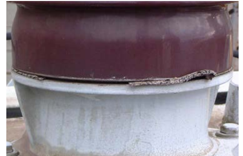
Figure 2. Compromised bushing gasket at flange-upper porcelain interface
