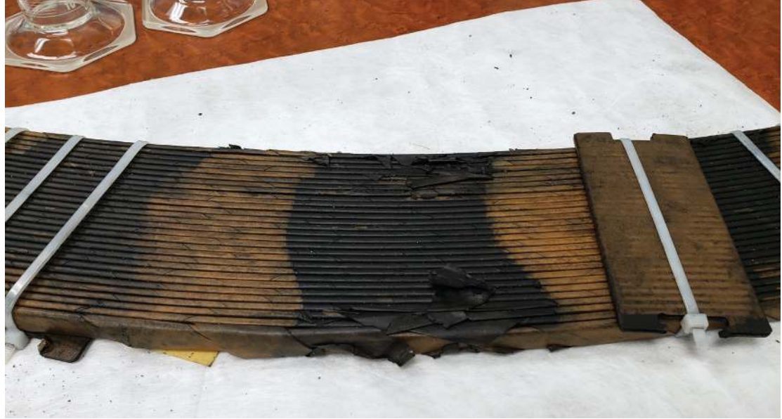
Figure 4: Example of Degraded Insulation
