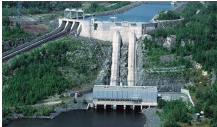
Lower Notch Generating Station Figure 2
