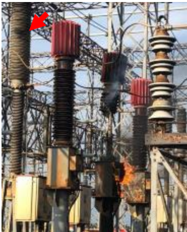
a) Failed CT in 161kV substation
