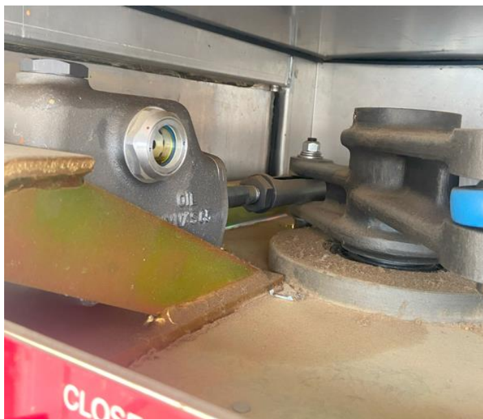
Example of Low Oil and Signs of Leakage Figure 9
