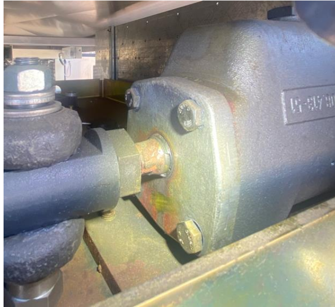
Compromised Shaft Seal Figure 5
