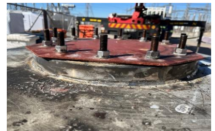
The Turret Where Welding Was Taking Place Figure 2c
