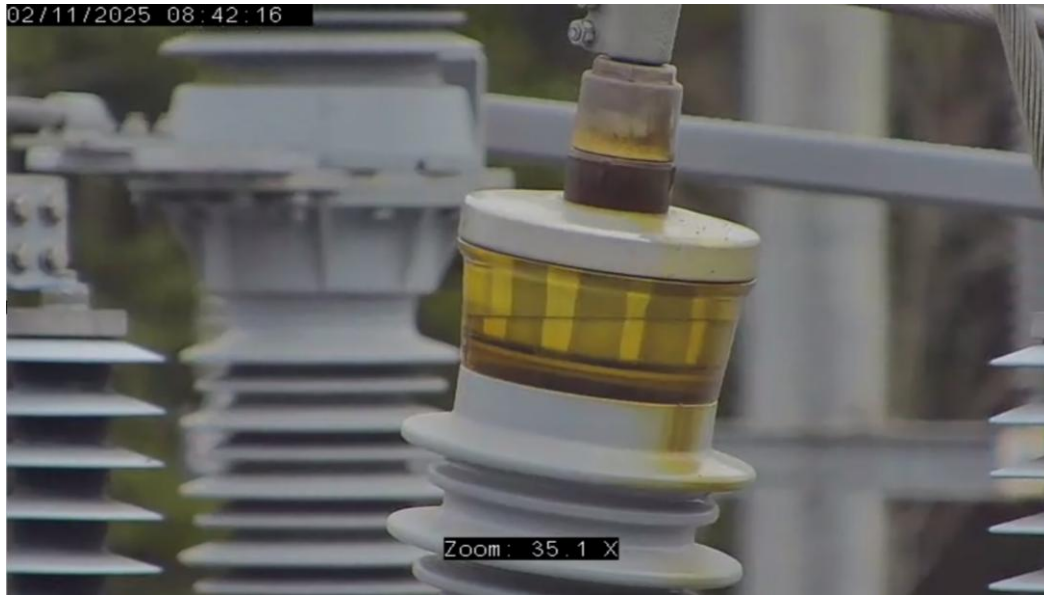
Image from Visual Camera Lens Showing Residue and Discoloration on Heating Bushing Figure 33
