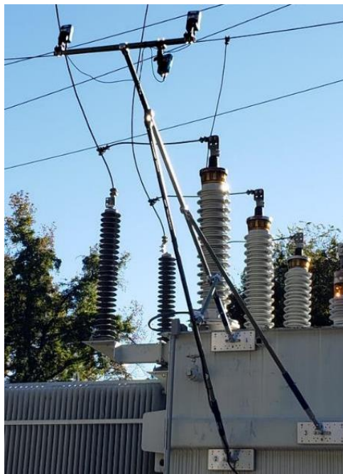
Example of Static Camera System Installation Figure 2
