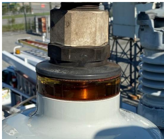
Image Showing Impact of Extreme Heat on Bushing Seals and Oil Figure 20
