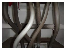
Figure 4 Lack of clearance between phases.
