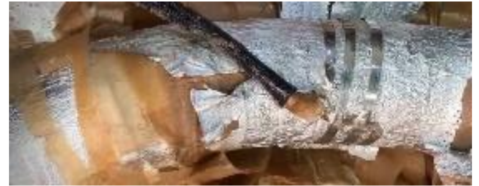
Internal ground connection
