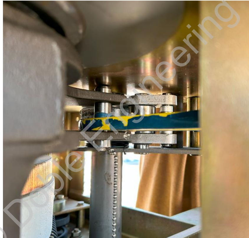
Slow Close Linkage Connection
