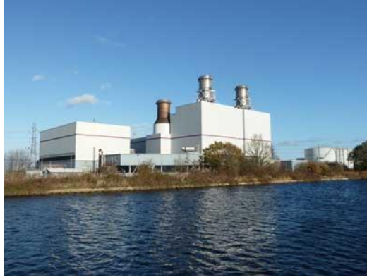
CCGT site in North Lincolnshire, UK used in this case study Figure 2
