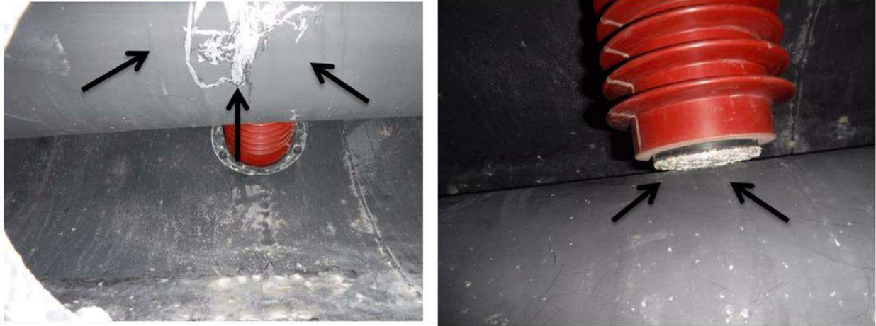
Inside the A phase of Unit 2 IPB; Evidence of PD was Found on both the Bus and the Insulator heads Figure 14
