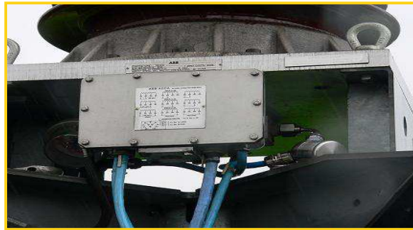
Figure 8 - Example of SF6 sensor application
