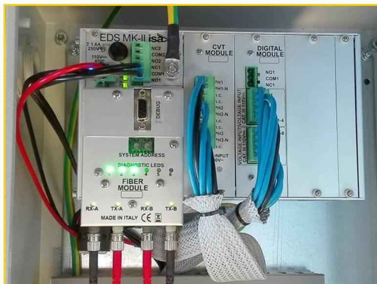
Figure 13 - Example of VTC Condition Monitor System 8 digital input
