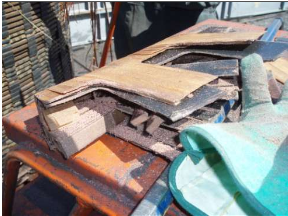
Case Study 2 – Over-wrapping from A Phase HV Winding FIGURE 10
