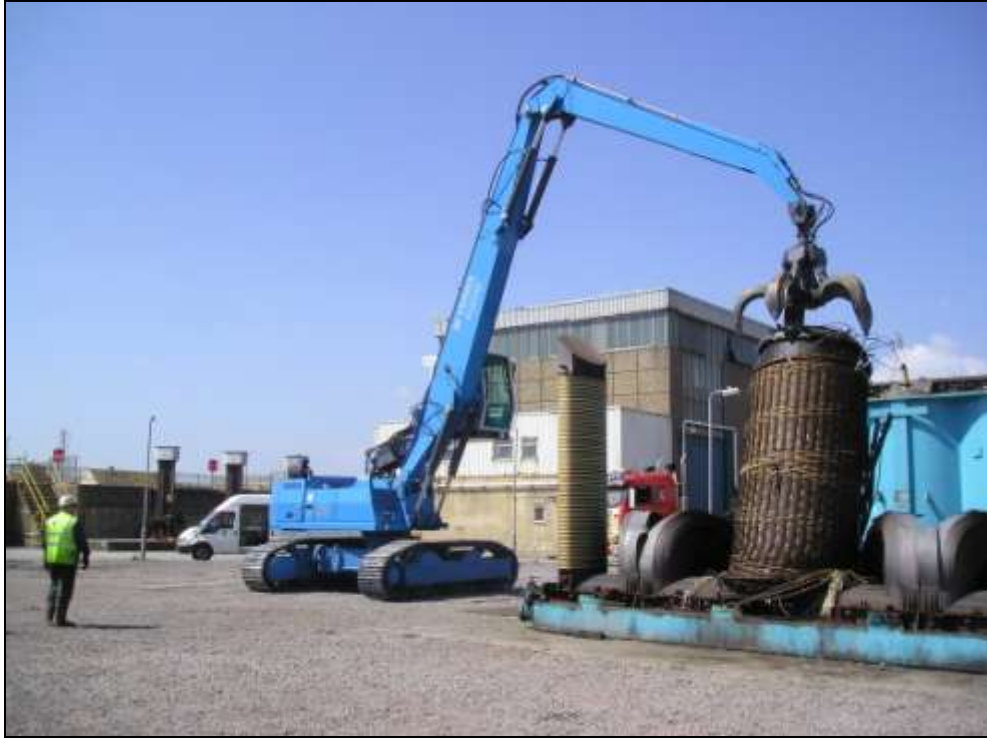
Case Study 2 – Scrapping Contractor Removing Damaged B phase Windings FIGURE 7
