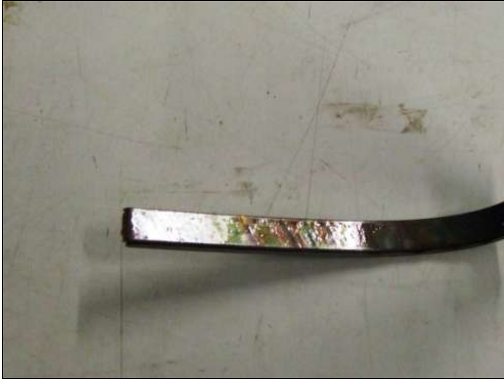
Case Study 1 – Sulphur Corrosion on Conductor from Top Disc of C Phase Series Winding FIGURE 3
