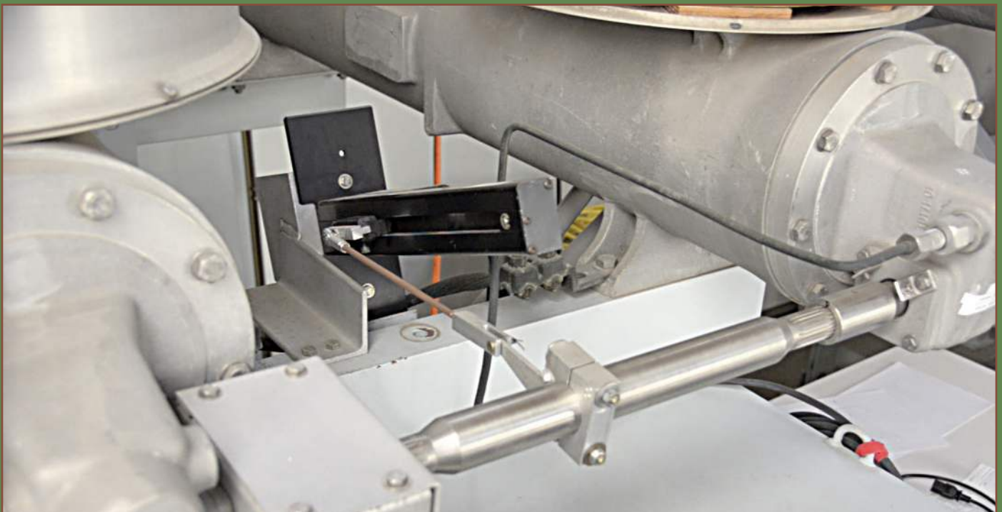
ABB 72PM Timing Rod Connected to Vanguard Linear Transducer
