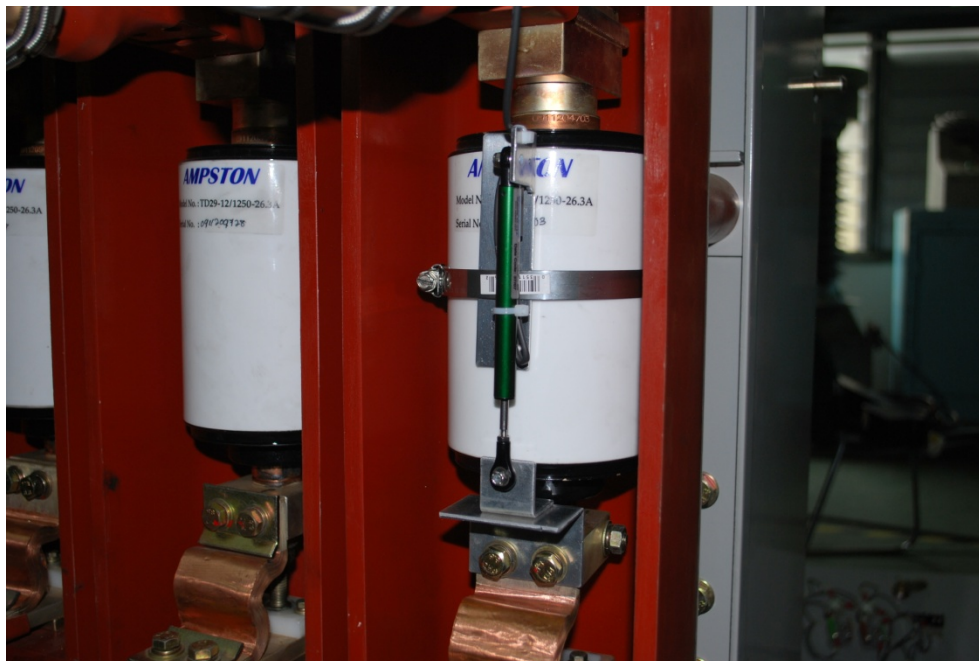
Resistor Transducer on Vacuum Circuit Breaker
