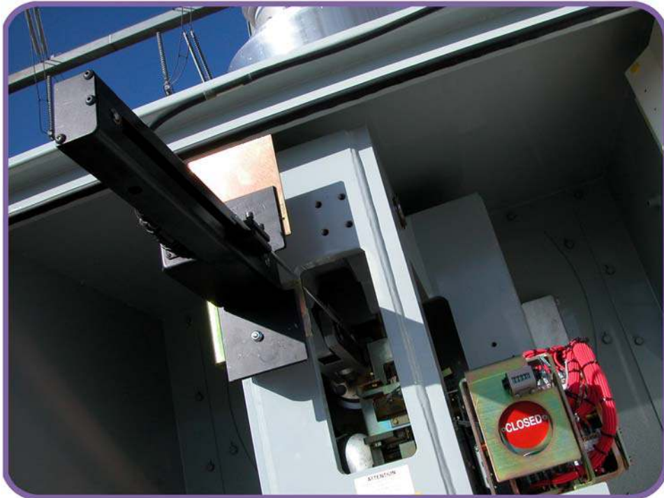
Figure 33. Linear Transducer on Mitsubishi 500-SFMT
