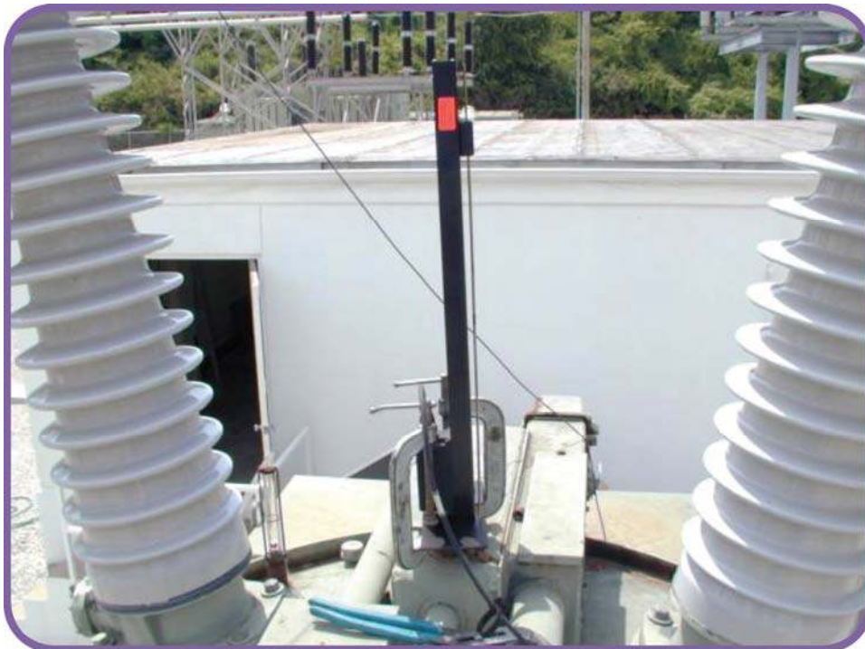
Figure 26. Linear Transducer on an OCB
