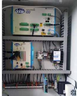
doblePRIME INSTALLATION In this example, this doblePRIME system includes a doblePRIME IDD and doblePRIME iO which are configured for true power factor with temperature compensation.
