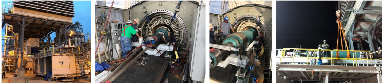
Generator Rotor Removal Figure 1
